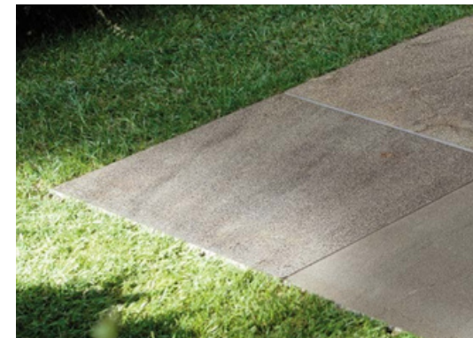
ADHESIVE INSTALLATION ON FOOTING
